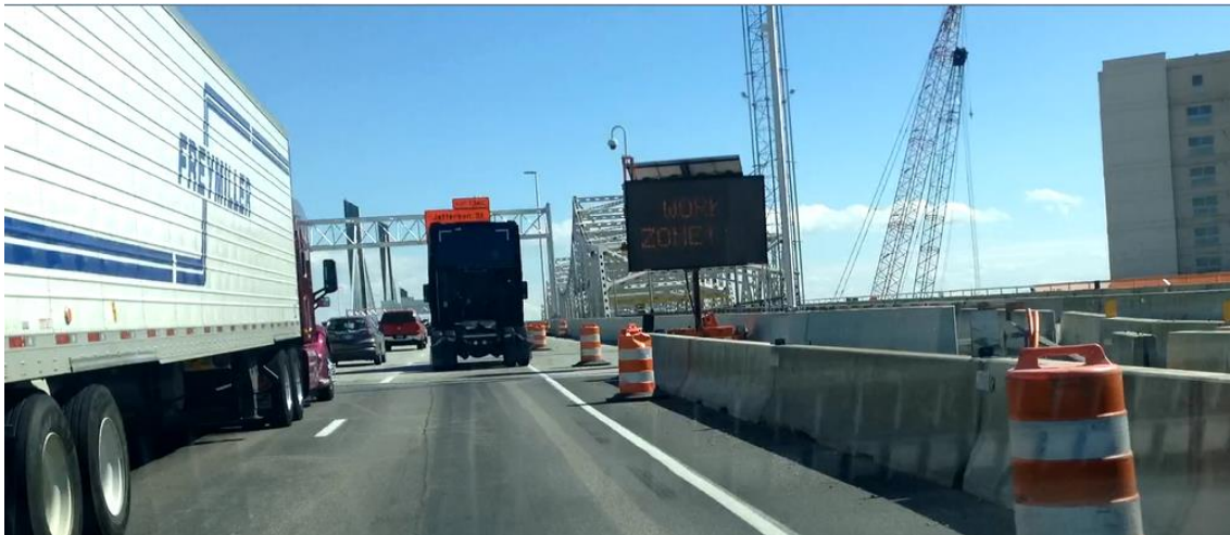
Figure 2: Construction Activity on Downtown Crossing
