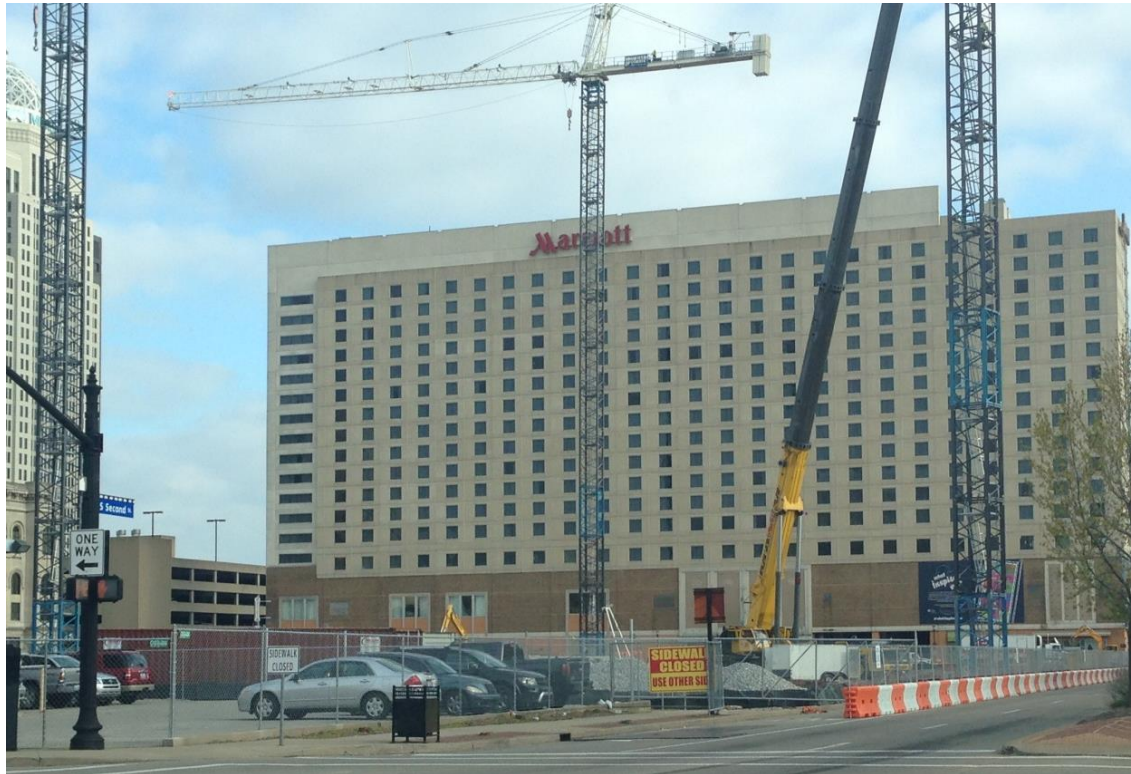
Figure 5: Construction Activity in Louisville
