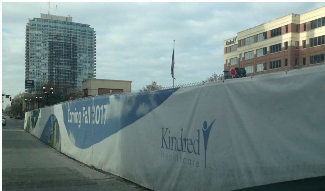
Figure 6: More Construction Activity in Louisville
