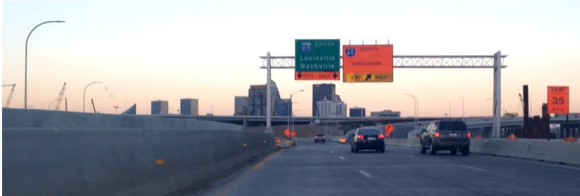
Figure 3: Construction Activity Near Downtown Crossing
